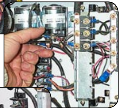
. . . pull wire out from opposite end. . .
