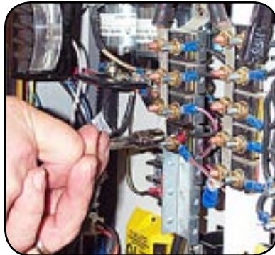
Install plain washer, lock washer, and nut. Tighten securely.
