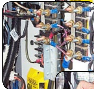
Install plain washer, lock washer, and nut.
