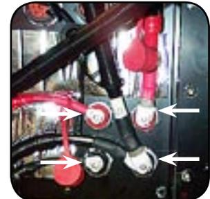
4 studs viewed from engine side of PDU panel
